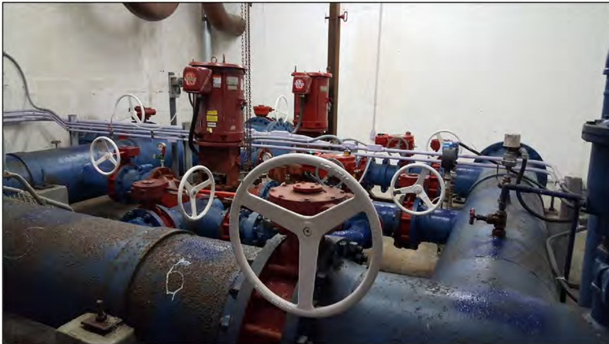
Exhibit 6.11: Corrosion on Piping
