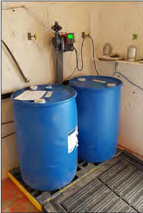
Exhibit 6.5: Small-Scale Sodium Hypochlorite System
