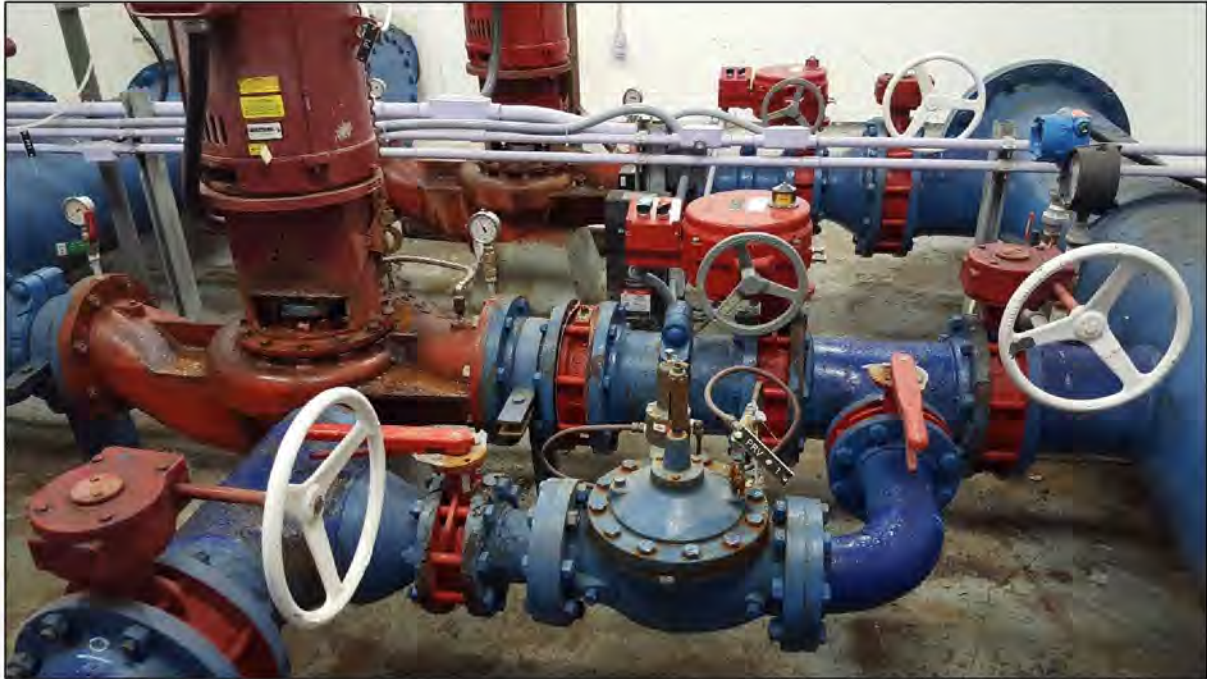
Exhibit 6.9: Visible Corrosion and Coating Degradation on Valves
