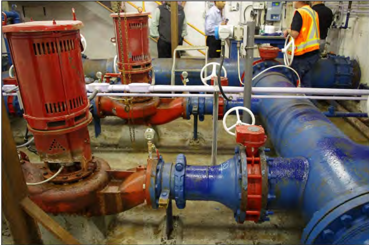
Exhibit 6.8: Visible Corrosion on Pump Casings
